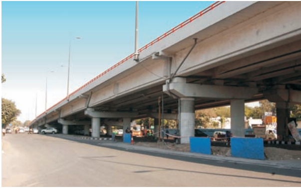
Flyover on NH2 connecting Faridabad
