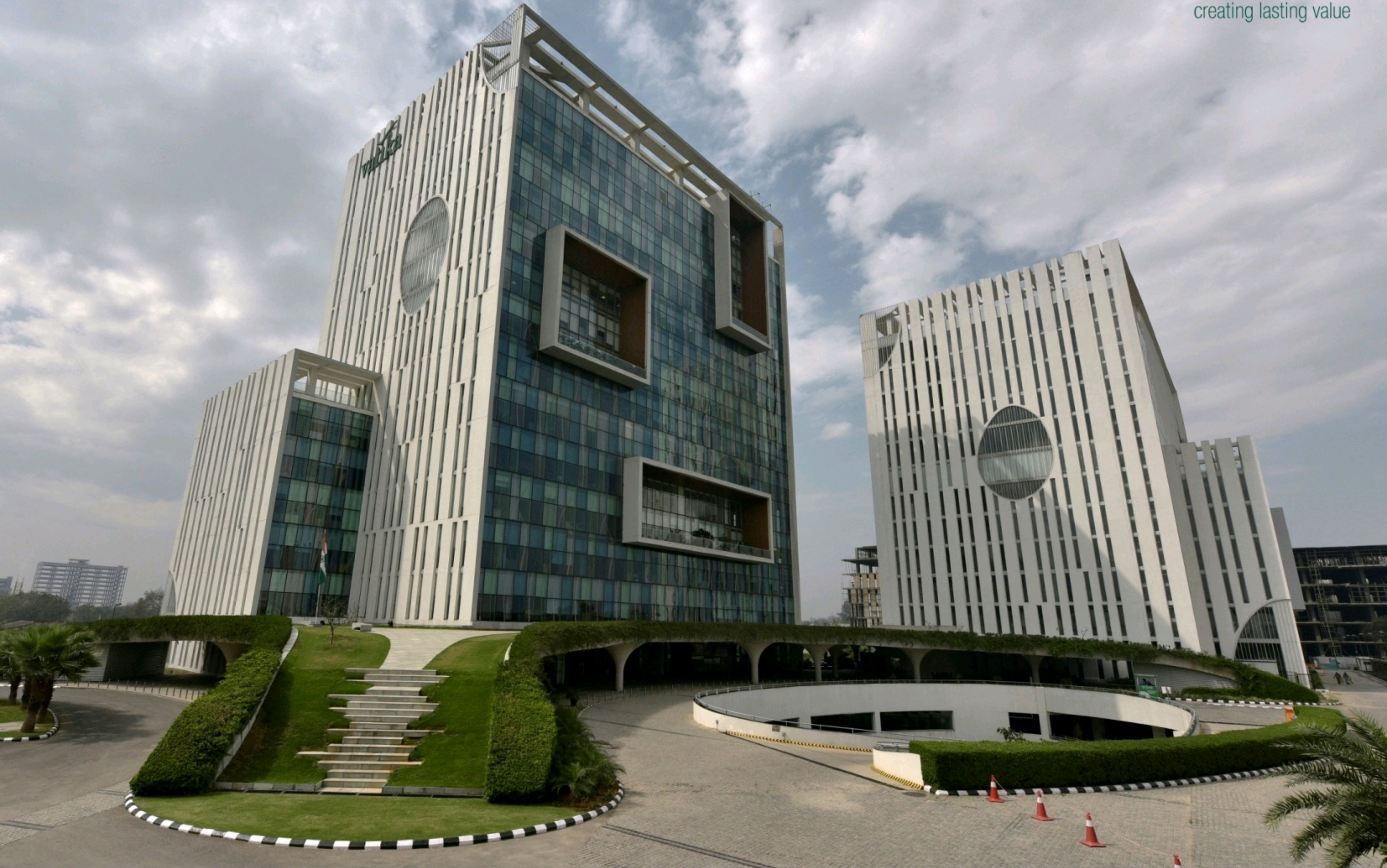
Entry to the complex and 1 st Floor Level – Walking Deck
